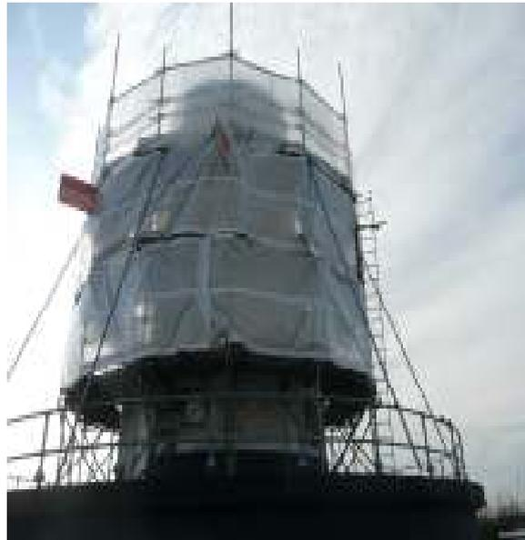
The Windmill Tower is still encased with plastic having been sand blasted to remove old paint and discoloration. The final cleaning and painting should be undertaken soon so that the Mill can be restored to its former glory. The trust has found it necessary to remove the sweeps, stocks and cap for this major overhaul.
